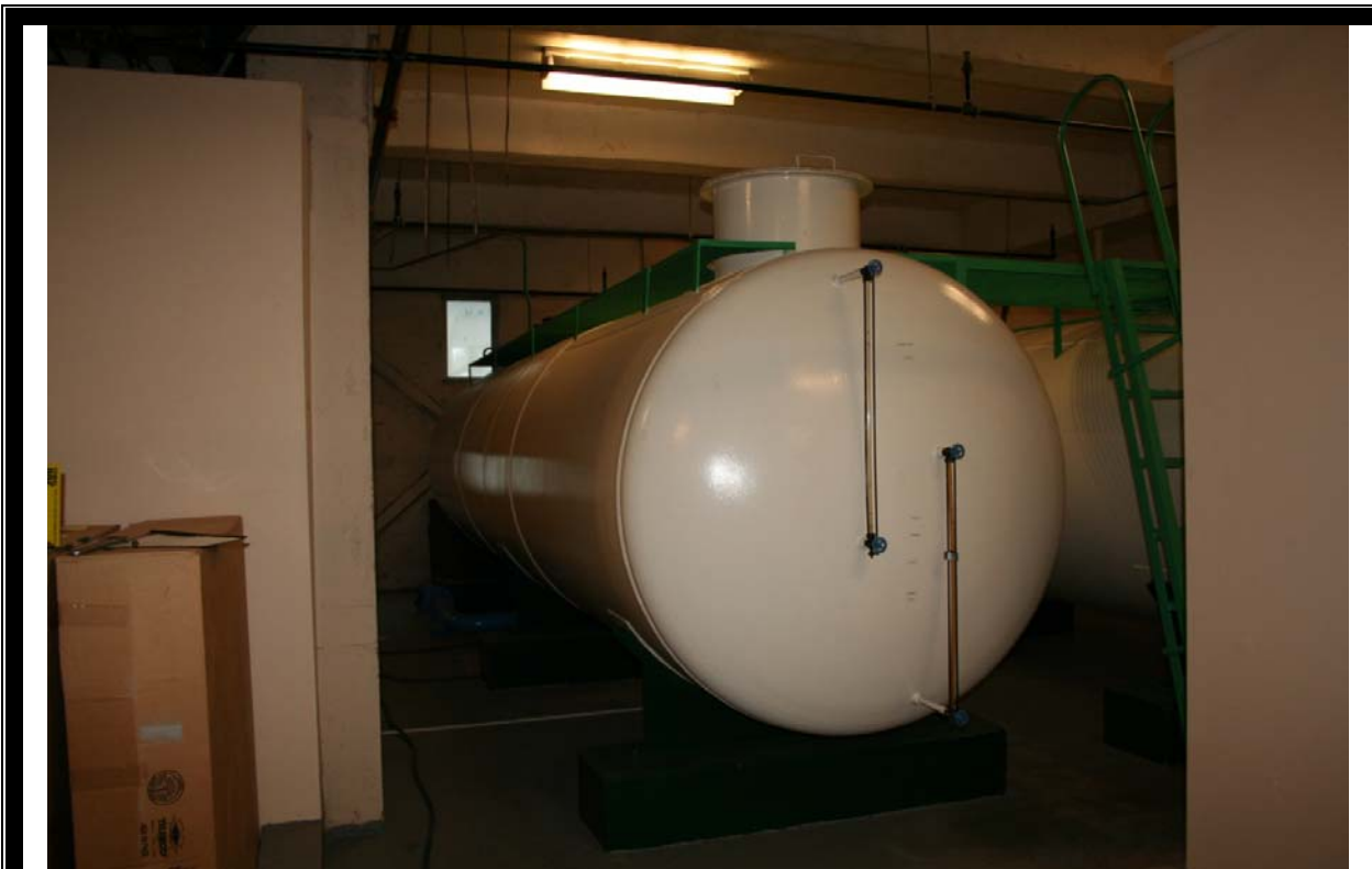
VIEW OF DOMESTIC WATER HOLDING TANK 6-23 FLOORS
